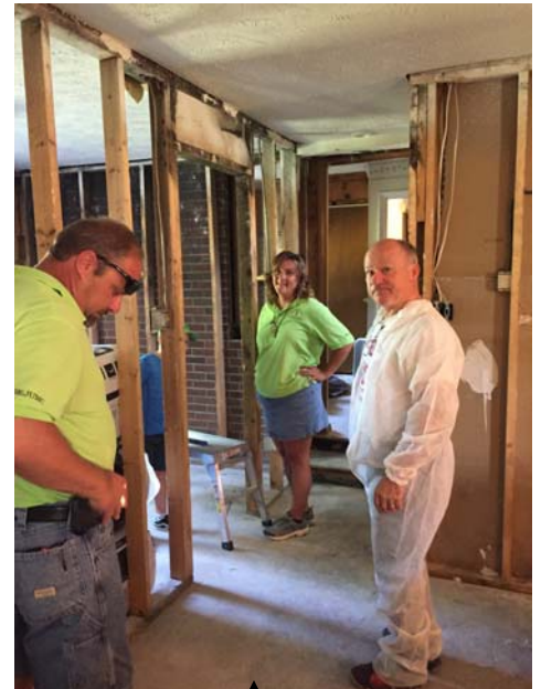
↑ Part of the inside crew with new studs & insulation in place
