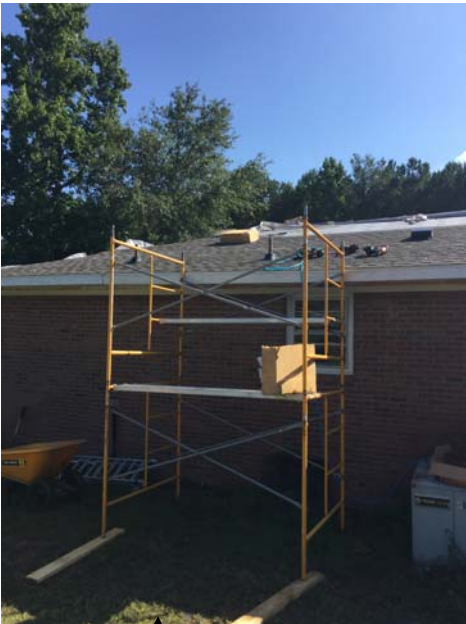
↑ New roof almost complete!
