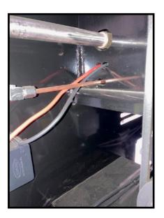
REPLACE WITH NEW PART AND THEN PROCEED TO FOLLOW THE 2 IGNITER WIRES INTO BURNER ROOM. CONNECT NEW WIRE TERMINAL.
