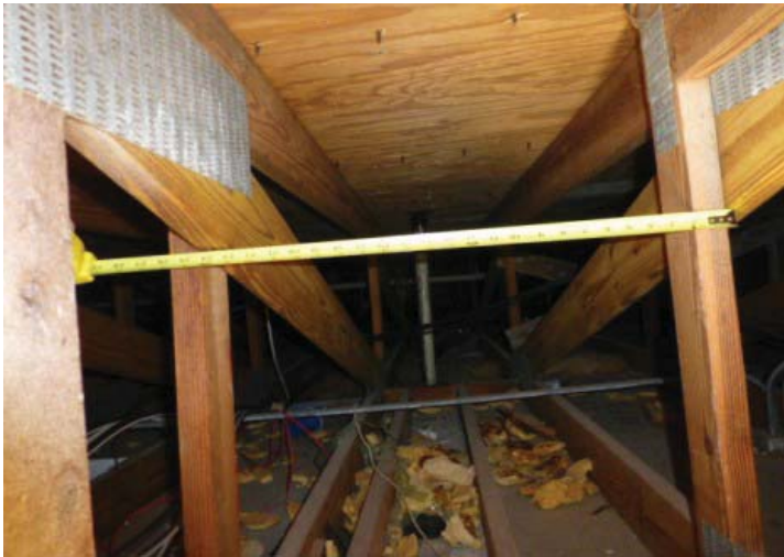
TRUSS/RAFTER SPACING
