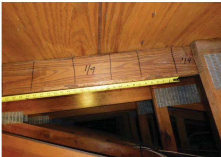
#3 ROOF DECK ATTACHMENT 6" X 6" NAIL SPACING
