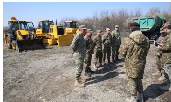
Military personnel from the 96 th Engineers Battalion during the hospital construction (Photo source: www.mapn.ro)
