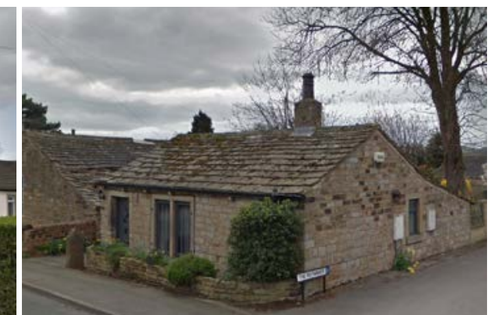
Single storey stone cottage conversion at junction with the Reynards
