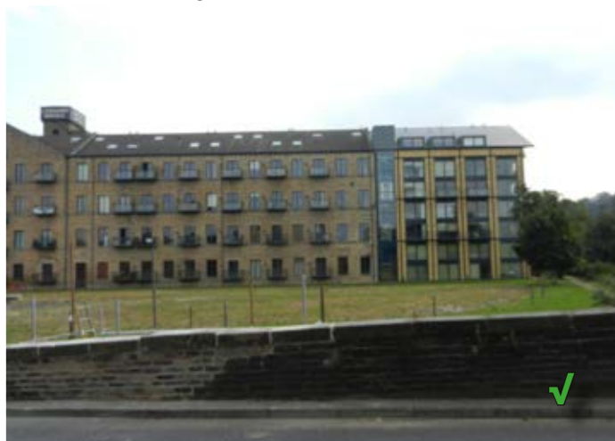
The extension to Ledgard Wharf is fittingly designed to relate to the proportions and materials of the original building but yet clearly expresses that it is a later addition through the glazed core that divides new and old.
