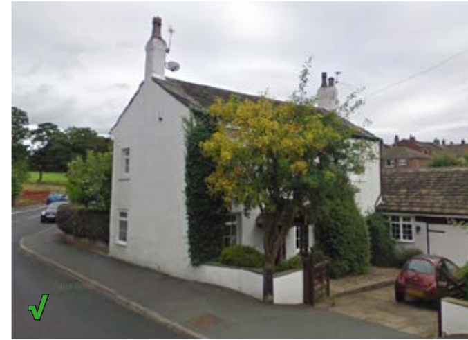
Cottage set at right-angles to the street
