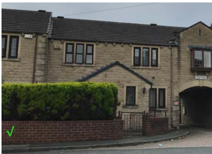
Wellhouse Court Mews is a modern take on a mews court typology with sympathetic detailing such as corbelling, stone window surrounds and rusticated stone
