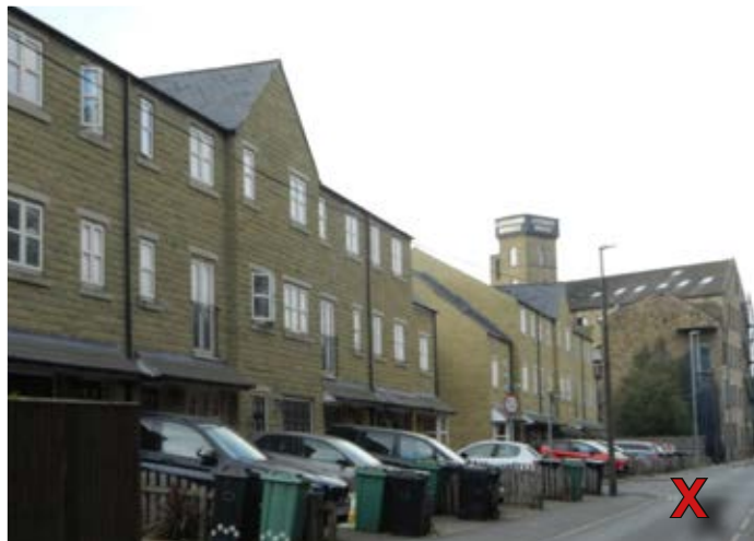
This combination front parking, bins and low quality boundary creates an unwelcoming and unattractive street scene that is unbecoming of what is otherwise a well considered townhouse development on Back Station Road next to Ledgard Wharf
