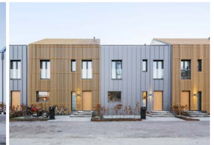
Figure 75: Cladding and roof angle varied to provide visual interest and aligned to north - south orientation
