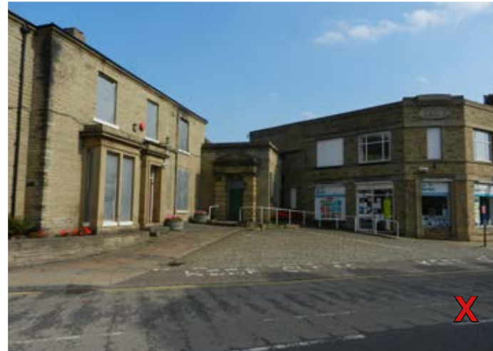
Boarded-up buildings detract from the environment and require bringing back into use, white painted railings and painted lines on the streetscape detract further overall
