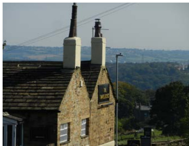
Figure 19: The Travellers Rest public house
