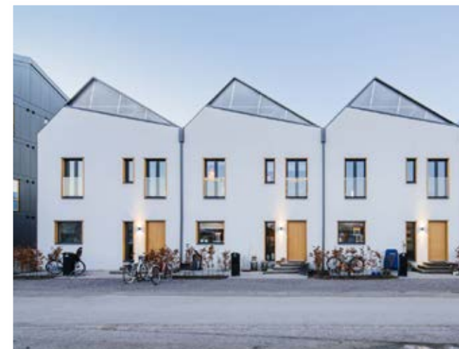
Figure 74: Asymmetrical roofs with photo-voltaics aligned for solar orientation in these 'solar terraces'
