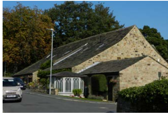
Figure 27: Main barn to Hall Farm
