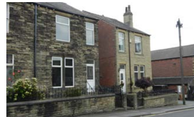
Figure 12: Example of typical street frontages in Mirfield
