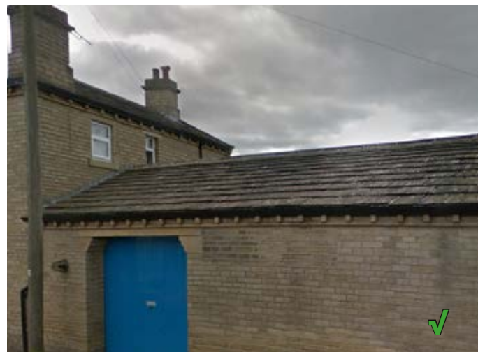
Single storey extension to building on Lee Green is subservient to the house and the detailing at the roof junction/eaves is good
