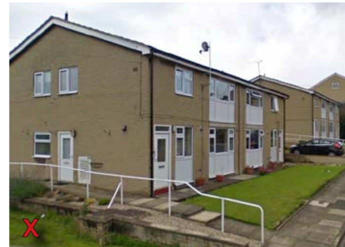
Later homes in Lower Hopton of a different scale, with different proportion windows and openings to the traditional terraces
