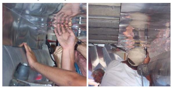
Mount sheeting with screws along floor joist / cross members moving towards center of boat where Water Glide will be mounted. **DO NOT PLACE SCREWS** to outer edge of sheeting where rails on Water Glide will be mounted.
