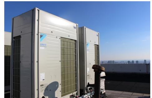
The Daikin VRV system is renowned for its efficiency, making it the ideal choice for multi-tenant buildings. Its capability to distribute refrigerant from the outdoor unit to multiple indoor units provides efficiency and reliability in one flexible package. The VRV equipment is modular and customizable, which was crucial to successfully meeting the challenges at Century Tower.
