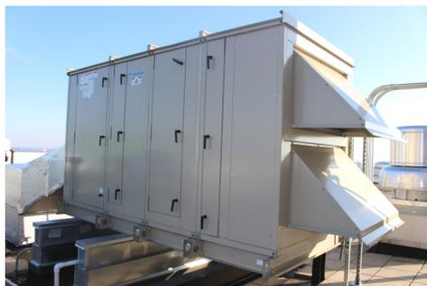
To the delight of Century Tower owners, D&B Building Solutions was able to provide a unique, state-of-the-art solution to accommodate their specific requirements. D&B supplied two Daikin Skyline Air Handling Units along with eight Daikin VRV Condensing Units, coupled together using an AHU integration valve kit. This innovative kit enables a non-VRV AHU to be seamlessly integrated into a VRV system, allowing the benefits of inverter technology to extend to all system components.
