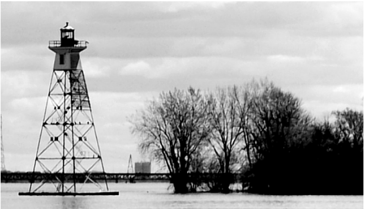
The Dixie Rear - replaced in 2019
