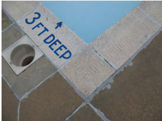
Photo 47 - Pool coping has been recently caulked
