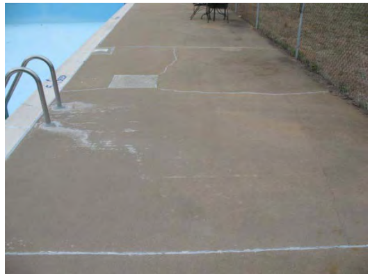
Photo 46 - Pool concrete deck
