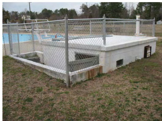
Photo 50 - Pool pump building has concrete block walls and concrete roof - roof should be periodically sealed against moisture
