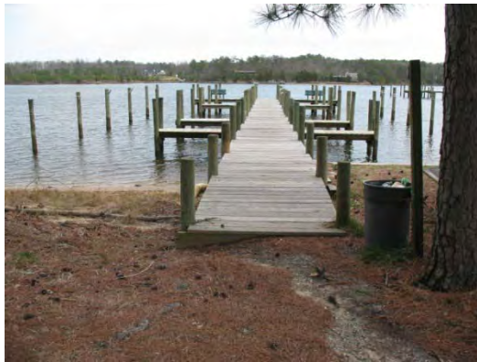
Photo 62 - View of pier and pilings
