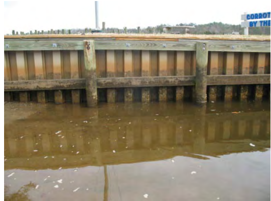
Photo 67 - View of bulkhead near boat ramp
