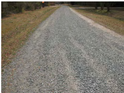
Photo 7 - Club View Dr. in good condition
