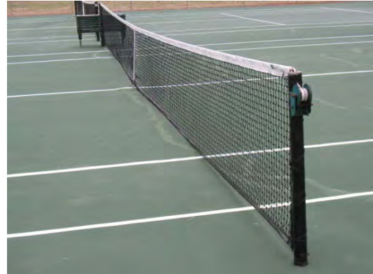
Photo 54 - Tennis court posts and nets in good condition
