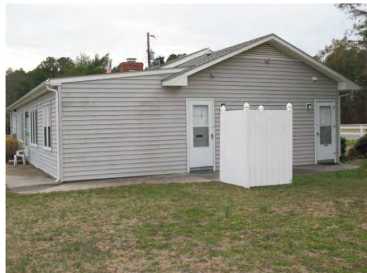
Photo 12 - Side and rear sidewalk at clubhouse
