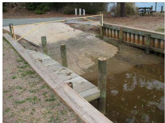
Photo 71 - Concrete boat ramp in good condition - Association plans to widen small area denoted by arrow
