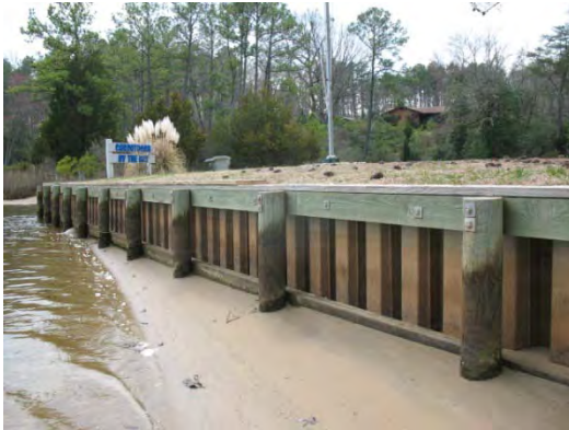
Photo 66 - View of bulkhead from pier
