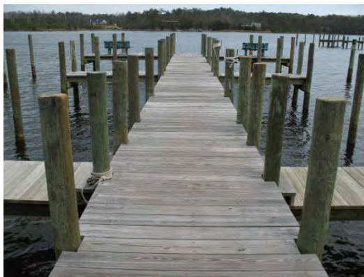
Photo 64 - Pier decking view
