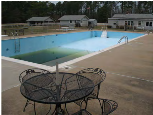
Photo 43 - Overall view of pool
