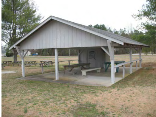
Photo 39 - Picnic shelter is in good condition
