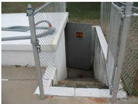
Photo 49 - Concrete steps down to pump room
