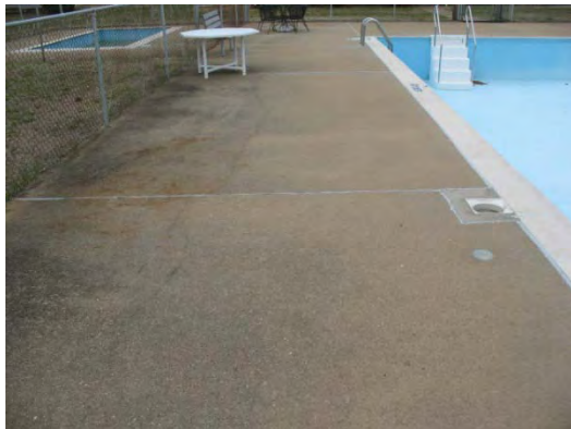
Photo 45 - Pool concrete deck
