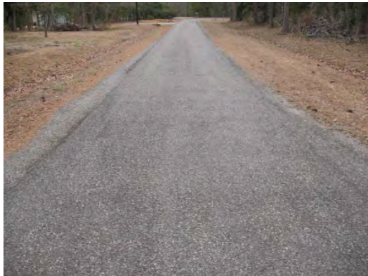
Photo 1 - Corrotoman Extension asphalt pavement in good condition
