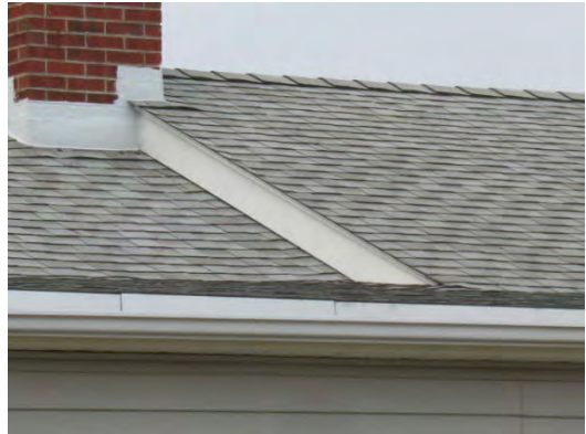
Photo 18 - Clubhouse rear roof view
