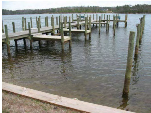
Photo 63 - View of pier and pilings
