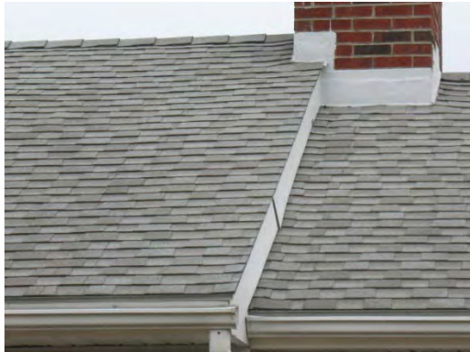
Photo 17 - Clubhouse front roof view
