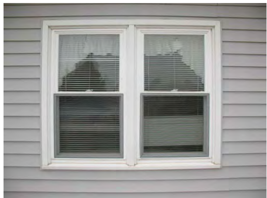
Photo 21 - Typical vinyl window
