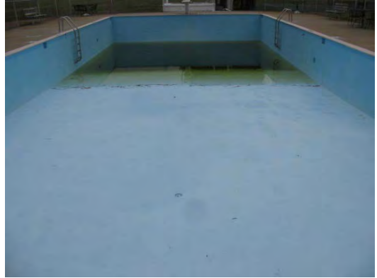
Photo 42 - Pool shell is painted annually
