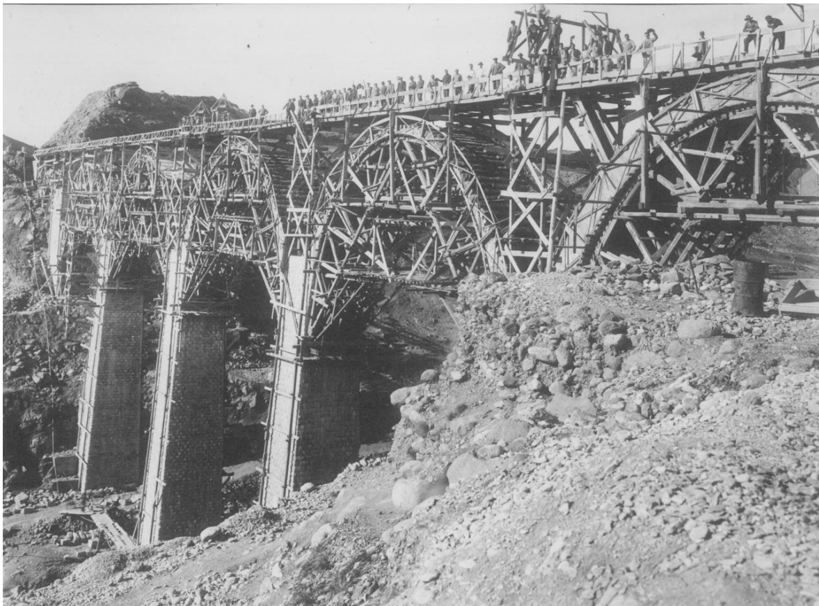
Costain built 11 miles of the Trans-Iranian Railway, seven tunnels and two viaducts in isolated mountainous terrain - for £1 million.
