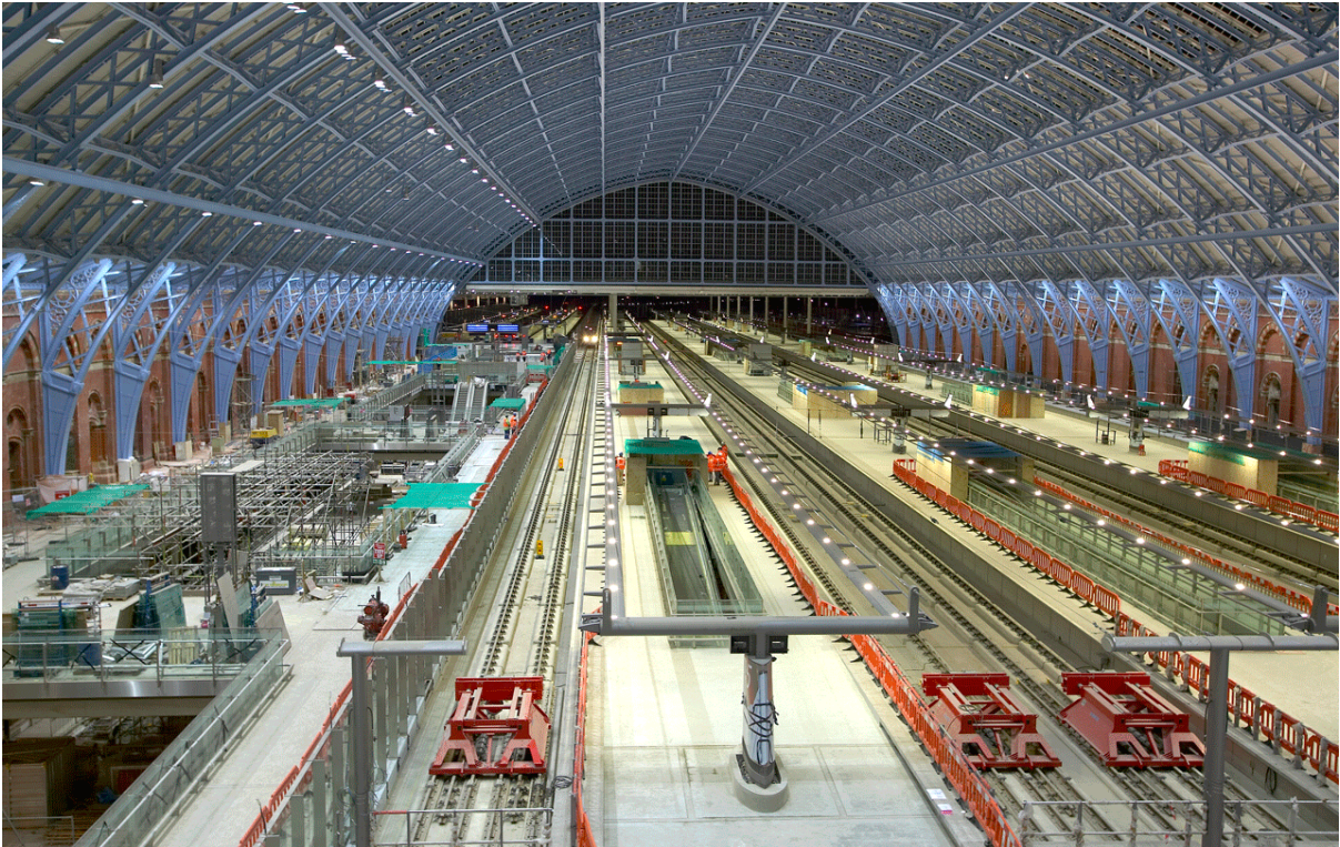
A Costain consortium completely restored London's St Pancras Station, in its time the world's largest single-span enclosed space.
