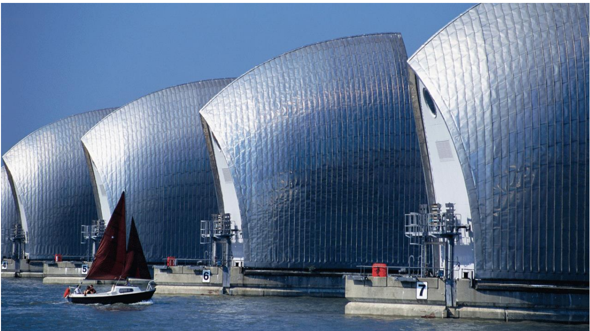
51,000 tonnes of structural steelwork and 214,000 cubic metres of concrete were used to build the Thames Barrier, on which Costain was lead contractor.
