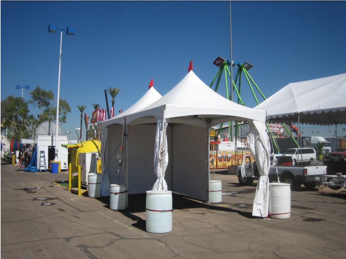
Two 10'x 10' tents with sidewalls secured with water barrels at the Arizona State Fair 2011
