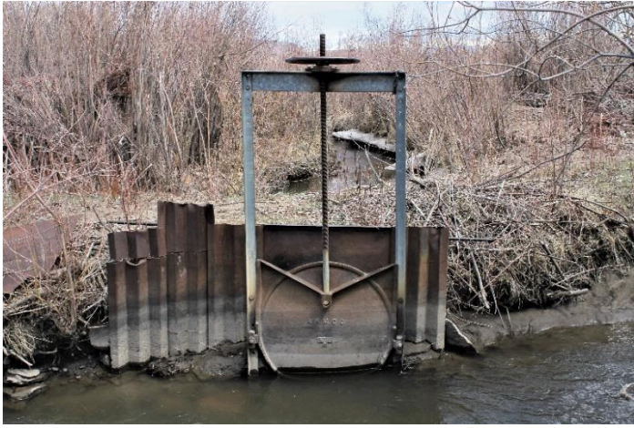
Headgate looking downstream
