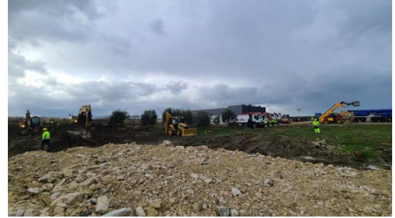
Works on Fier hospital have started (Photo source: www.kryeministria.al)
