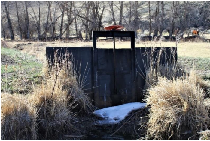
Headgate looking downstream
