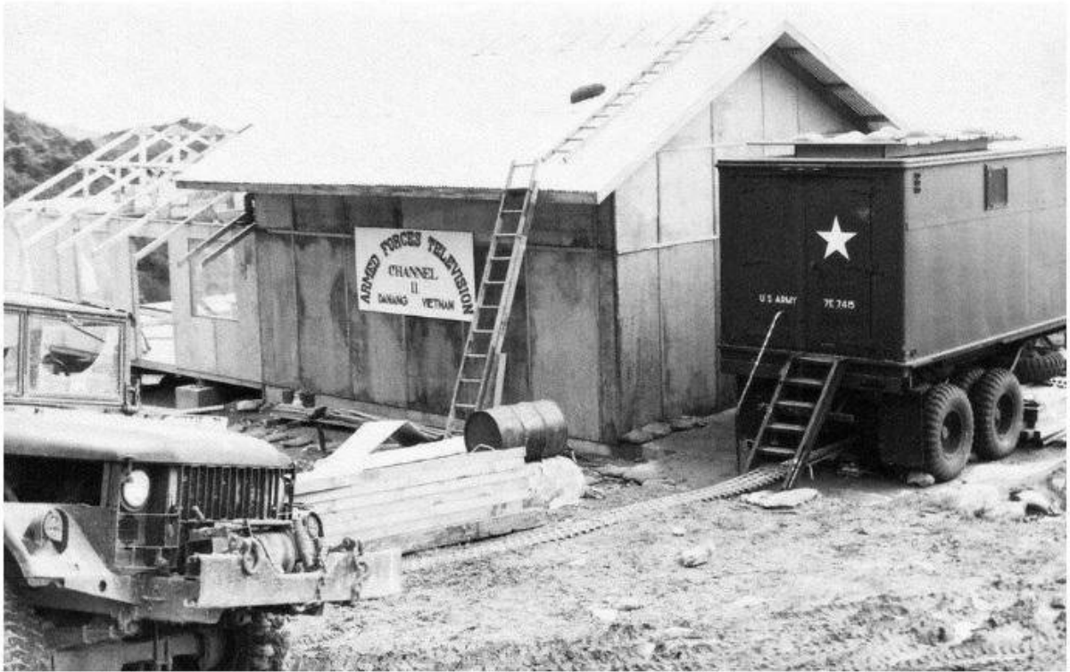
Construction of Detachment 2, Da Nang.
