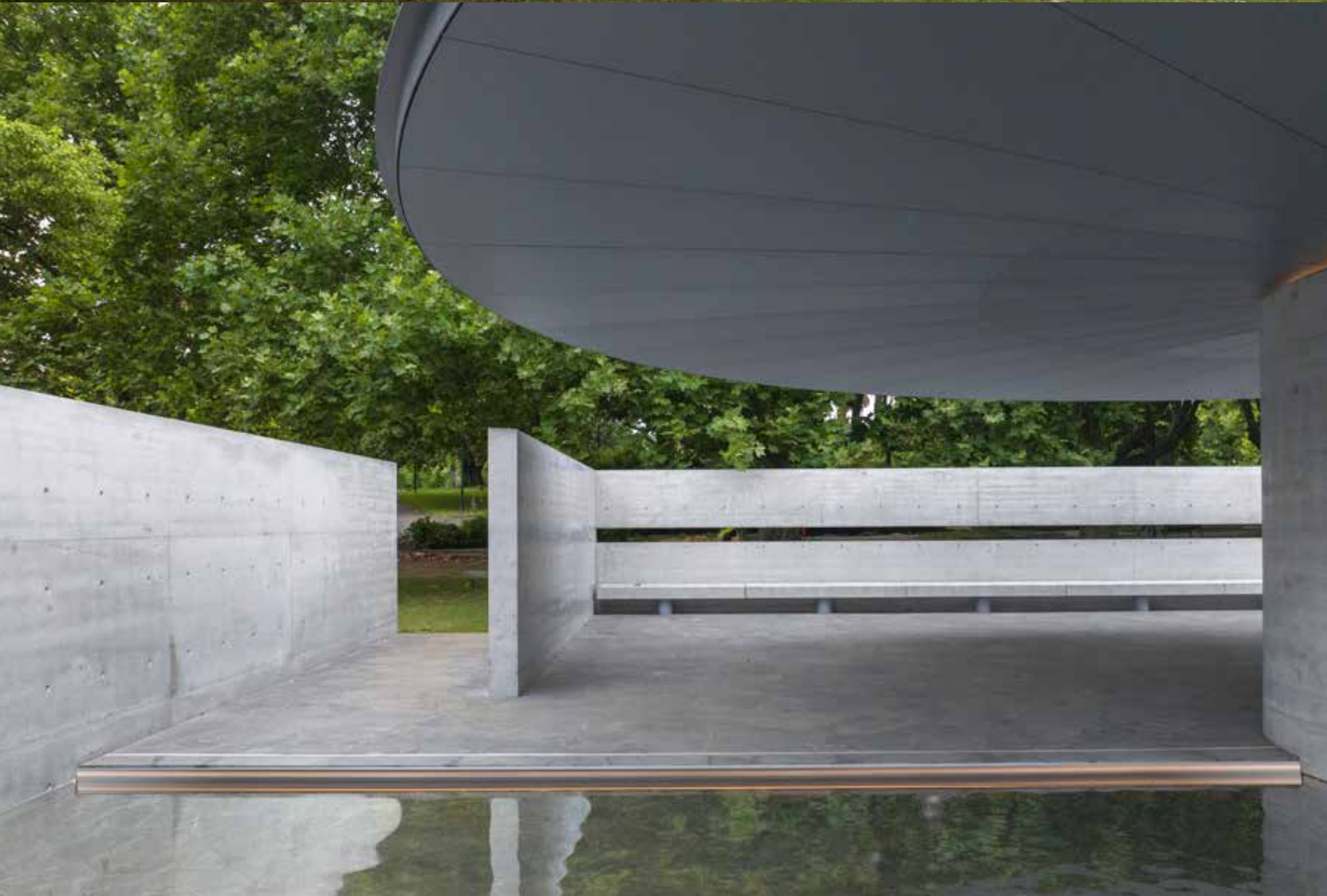
The walls of the pavilion are reinforced self-supporting concrete. (Below) The reflecting pool mirrors the canopy, sky, city, and surrounding nature.
