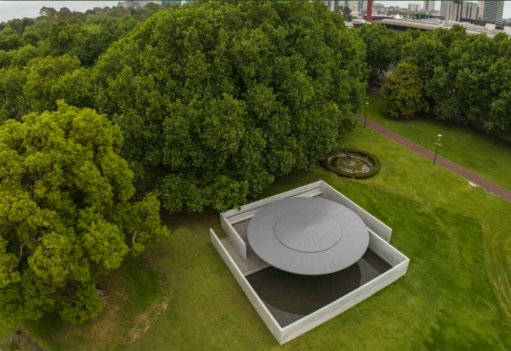
A horizontal opening runs the length of the north and south walls. (Below) Two offset squares create two entrances that lead to the centre of the pavilion.
