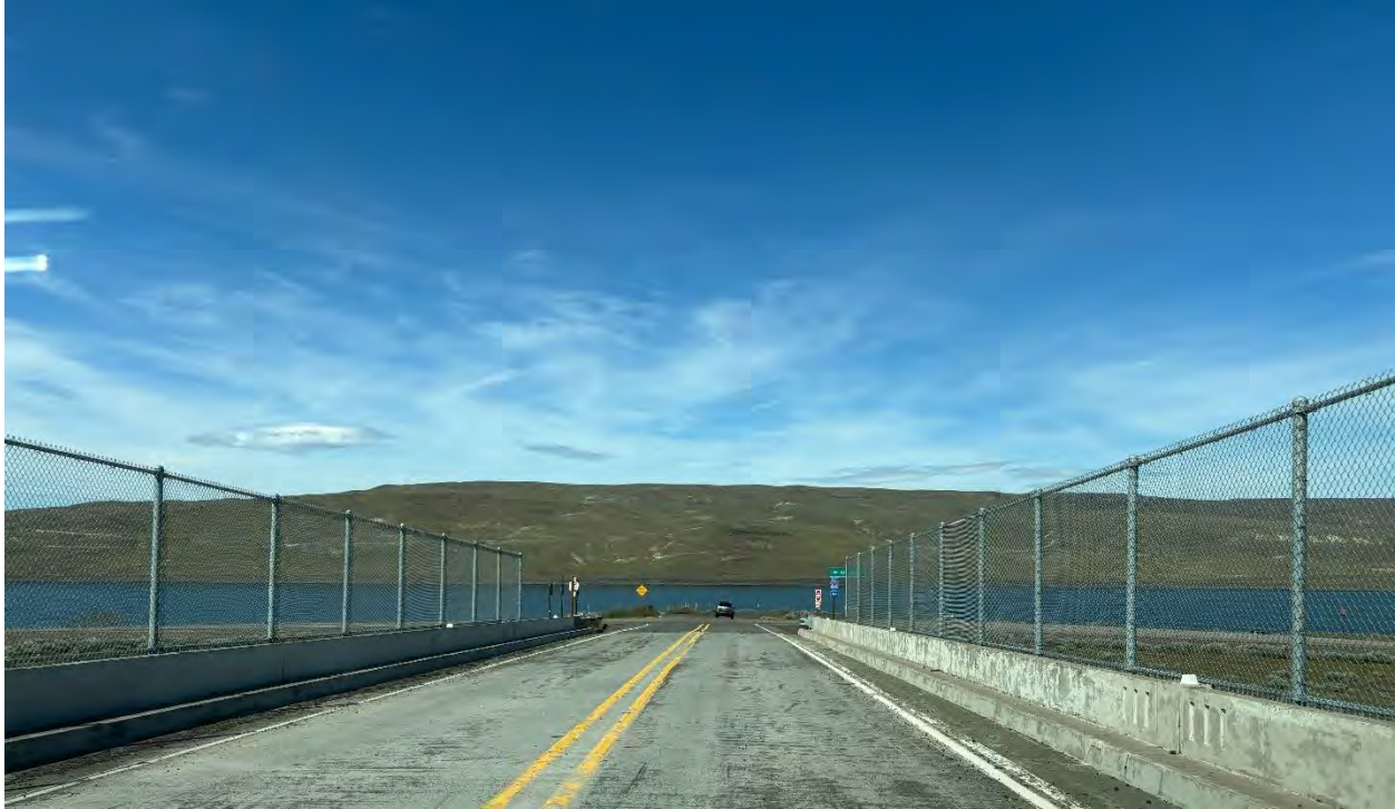
Figure 2.3: Willow Creek Site Access Bridge
