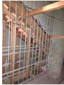
Formwork & safety shoring
