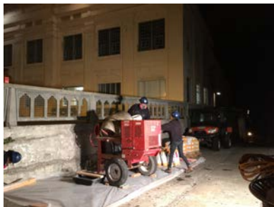
Concrete mixer; repairs completed at night to avoid visitor interruption
