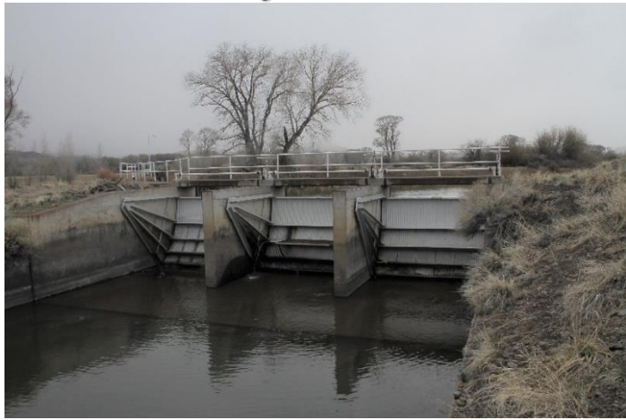
Leaking headgate
