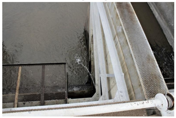
Leaking headgate
