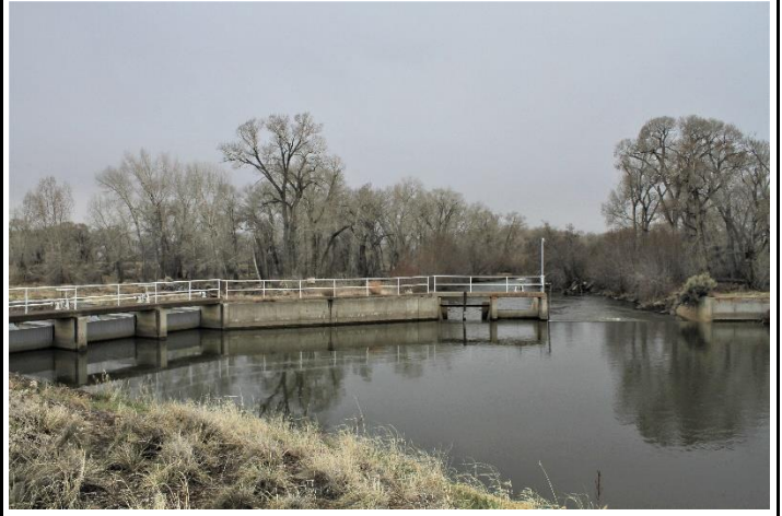
Headgate and diversion dam
