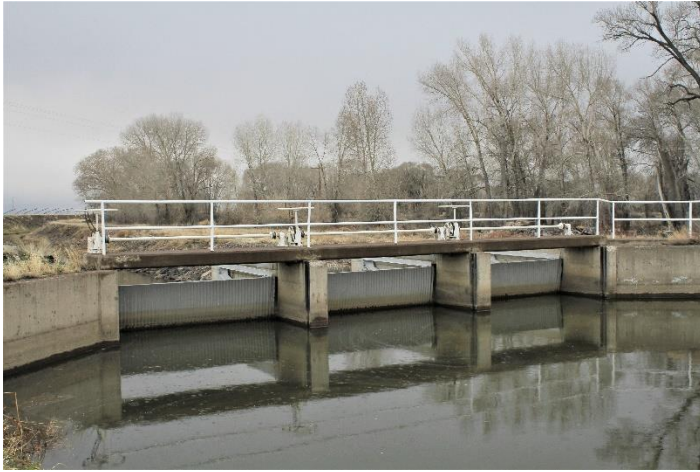
Headgate looking downstream
