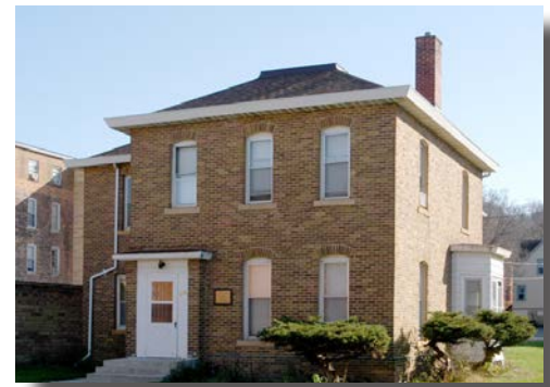
315 South Broad Street
