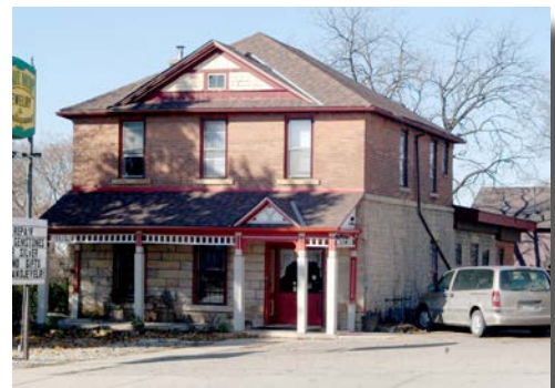
Stone structure at 816 North 2nd Street
