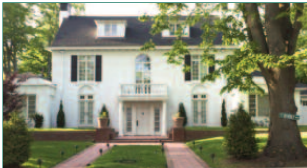
17 Beverly taken in 2017 after four years of restoration
