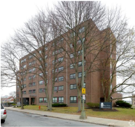
Boa Vista Tower's High-Rise Building
