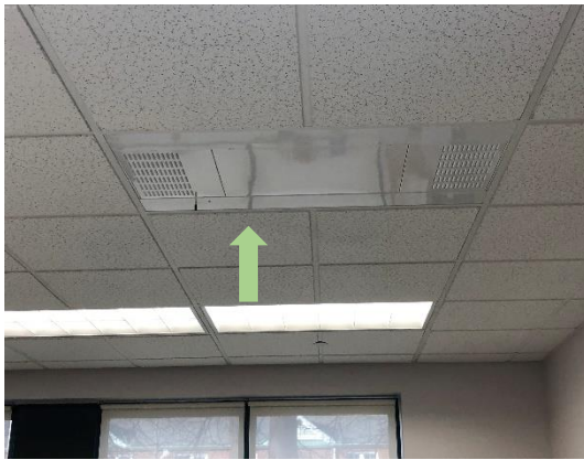
BOA Vista Towers office space installation
