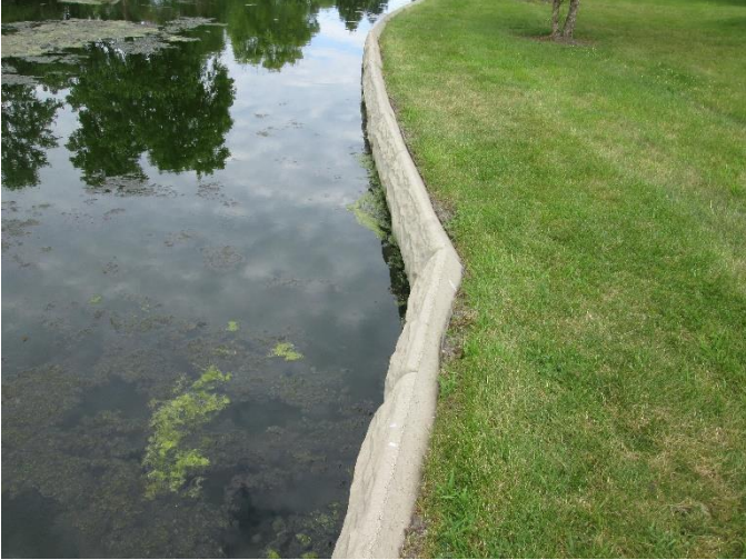
Channel lined with large concrete retaining wall blocks
