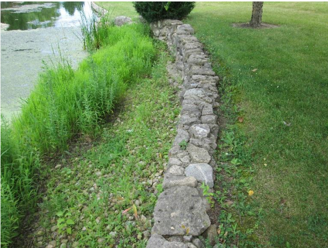
Western portions of channel are lined with stone retaining walls
