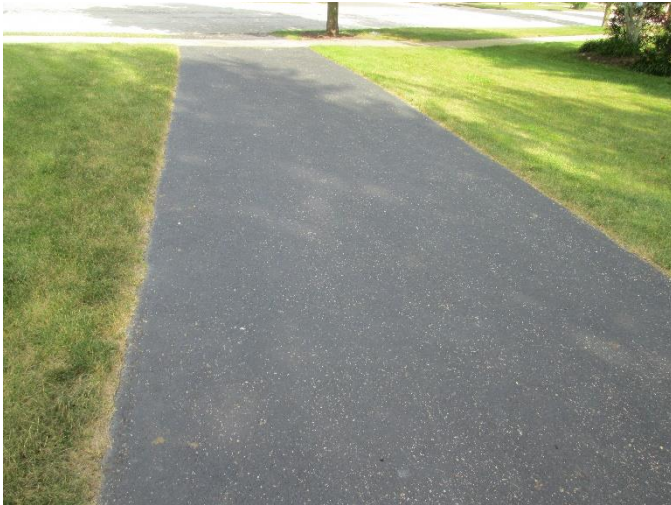
Asphalt pavement service drive near west tennis court
