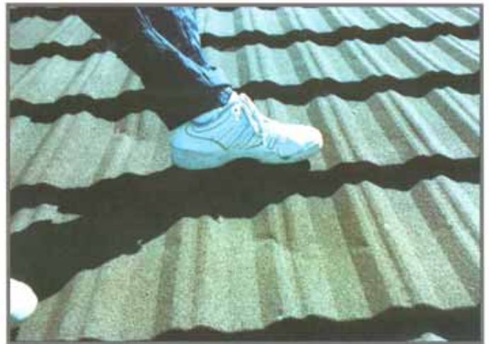
Proper foot position on metal tile panels.
