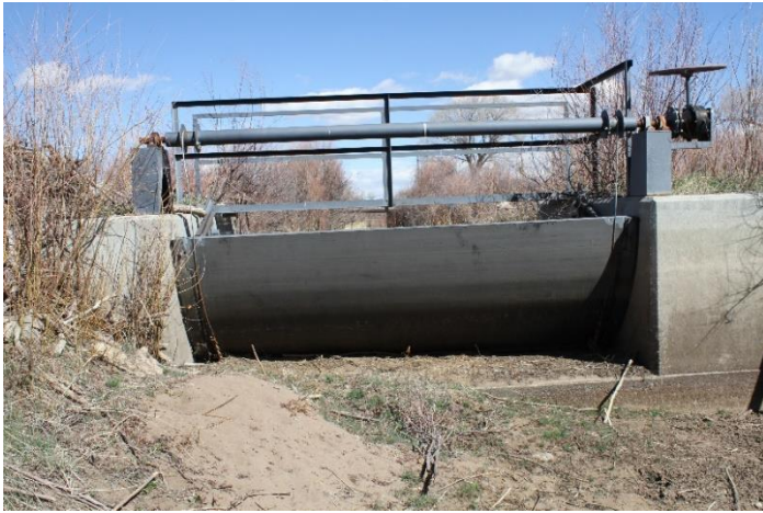
Headgate looking downstream
