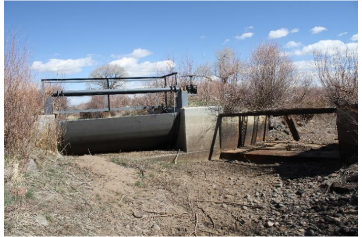
Headgate and diversion structure
