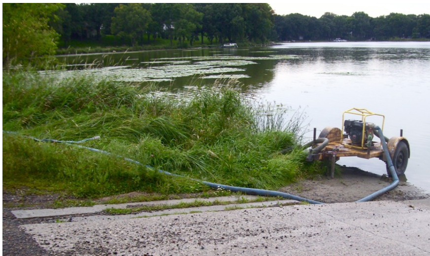
The HARDDRIVES pump placed at the Rush Lake Access to provide water to control the dust from the County Road 16 resurfacing project.
