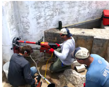
Horizontal core drilling for material testing
