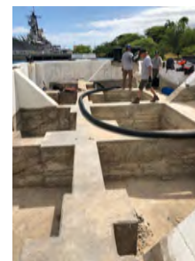
Exposed structure after sand removal
