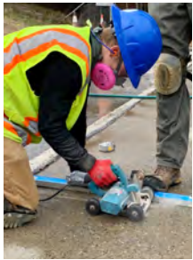
Saw cutting expansion joints on hardened concrete
