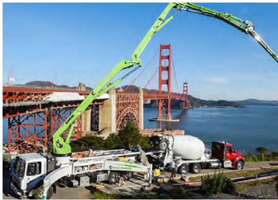
Ready mixed concrete truck and pump setting up just after daybreak at project site
