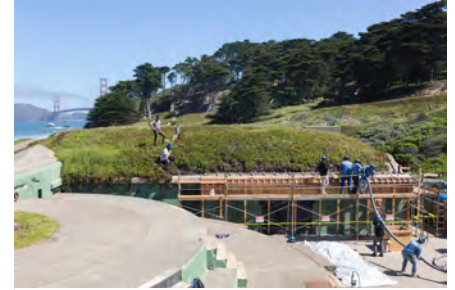
Work site; Golden Gate Bridge in background
