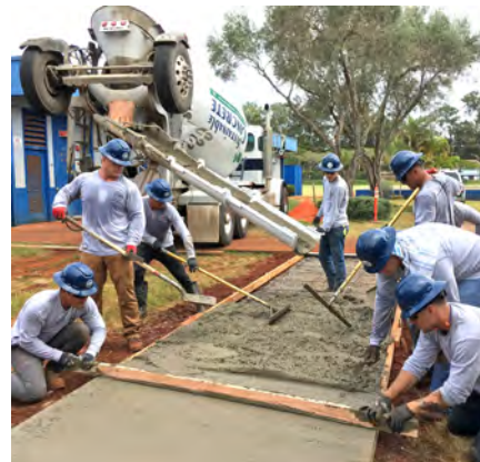
In Progress: Placing concrete
