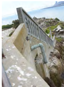
Completed stair railing from cliff side
