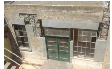
Historic window and doors reinstalled integrally with façade concrete
