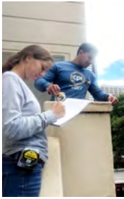
Assessing conditions, planning repairs
