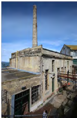
Before: Power House
