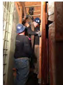
Moving concrete-loaded hose to next port during high-pressure pumping
