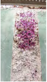
Concrete carbonation testing
