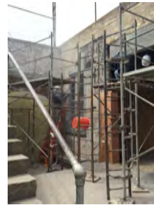
Scaffolding constructed by team at facade
