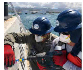
Concrete drilling to collect samples for chloride testing
