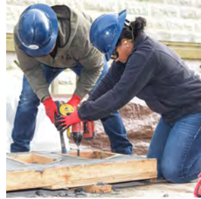
Removing formwork from completed precast panel
