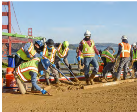
Placing & finishing pumped concrete
