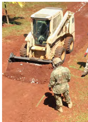
In Progress: Site preparation
