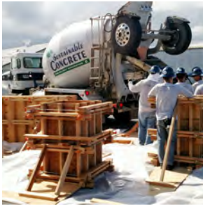
Pre-project formwork and ready-mix concrete training
