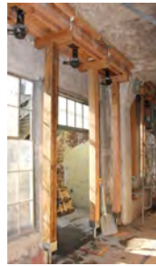
Interior façade beam formwork
