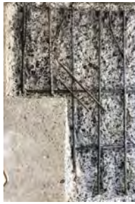
Partial depth slab repair: concrete removal; reinforcing hand placed placement
