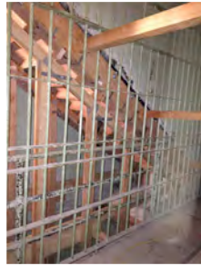
Formwork & safety shoring
