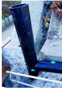
New drainage pipe installed, later embedded in concrete
