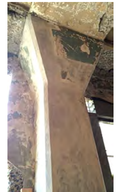
After: Interior column with preserved historic material, prior to painting
