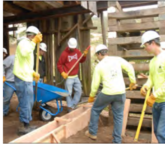
Foundation concrete placement
