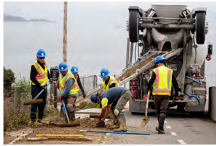
Placing truck discharged concrete
