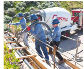
In Progress: concrete placed via pressure pumping
