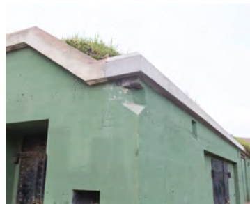
After: Repairs complete
