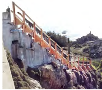
CPI constructed safety railing in place during project
