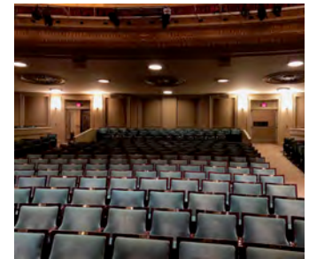
Repaired door surrounds at back of theater
