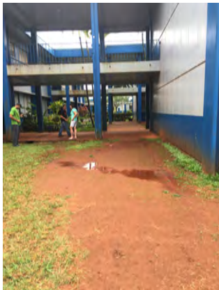
Before: Red clay dirt/mud at entrance
