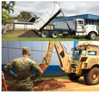
Top & Bottom: Managing heavy equipment work
