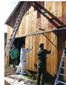
Painting repaired barn with NPS staff
