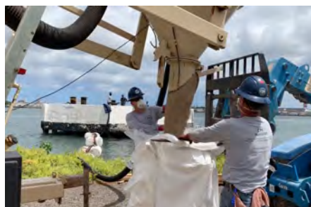
Pumping sand ballast out of mooring structure to allow inspection/repair
