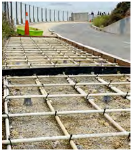
Site prep & glass fiber reinforcing bars installed
