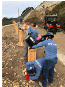
Constructing walkway at base of stairs
