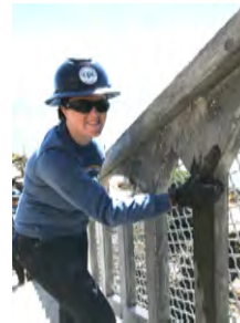
Installing welded wire mesh for visitor safety
