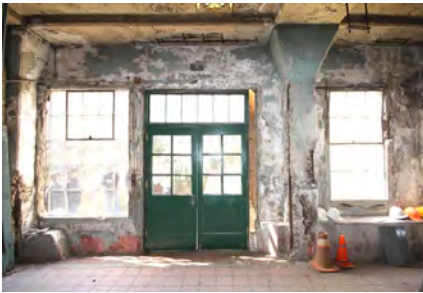
Interior façade existing conditions
