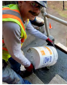
Partial depth slab repair concrete hand placed
