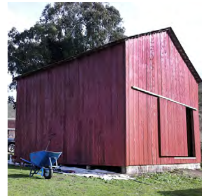
After: Repairs complete, building rear
