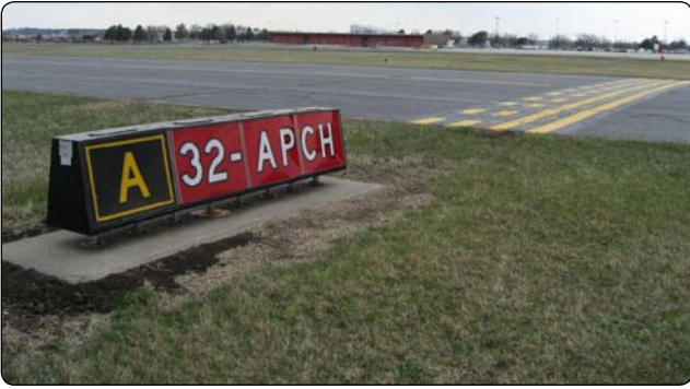
Figure 1-37. Runway 32 approach area sign and marking on Taxiway Alpha.
