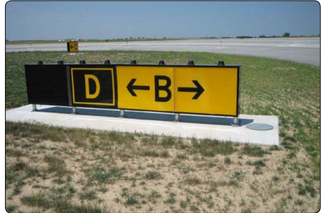
Figure 1-31. Taxiway Bravo direction sign with a collocated Taxiway Delta location sign. When the arrow on the direction sign indicates a turn, the sign is located prior to the intersection.
