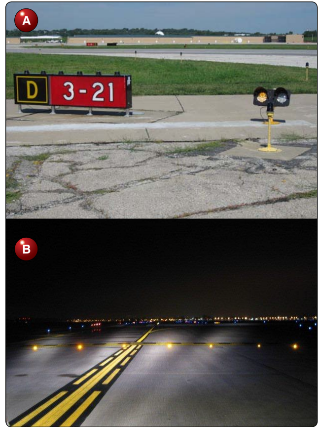
Figure 1-26. (A) Elevated flashing yellow runway guard lights also referred to as “wig-wag” lights. (B) In-pavement flashing yellow runway guard lights.
