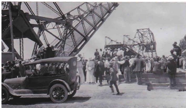
The deck was wooden and became heavy when sodden with rainwater. To counterbalance this weight, extra concrete blocks were seasonably added to the huge concrete counterweights. A sidewalk on the downstream side was added after several vehicle-pedestrian accidents occurred on the bridge. Funds to add the walkway were raised by the Delta Progress Club and the Walnut Grove Boy Scouts.
