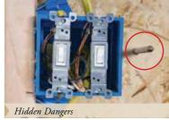
Nails that miss their mark can be potentially hazardous to items, like wiring and plumbing, located in the cavities between studs.
