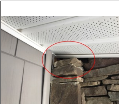
An opening above the veneer stone should be sealed as necessary.
