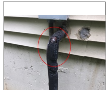
Damage / missing refrigerant line insulation.
