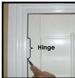
Mark should be made on the wall/jam at the bottom of the hinge.
