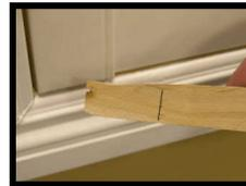
*Tip: The shim that is marked with a pencil, can be used as a guide for the right panel height spacing.*
