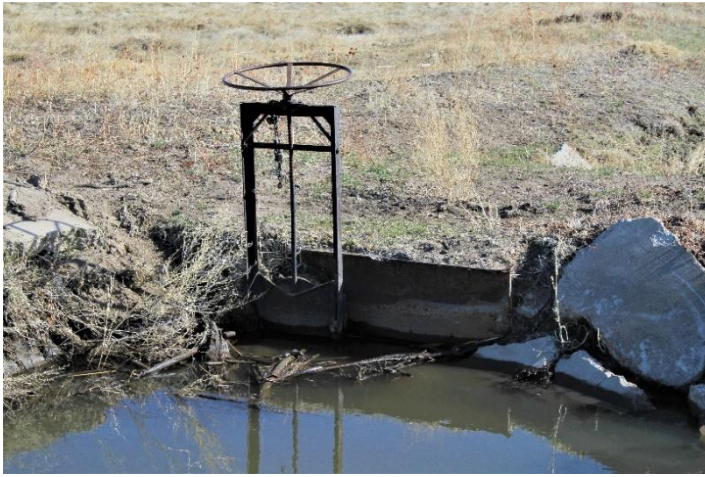
Headgate looking downstream
