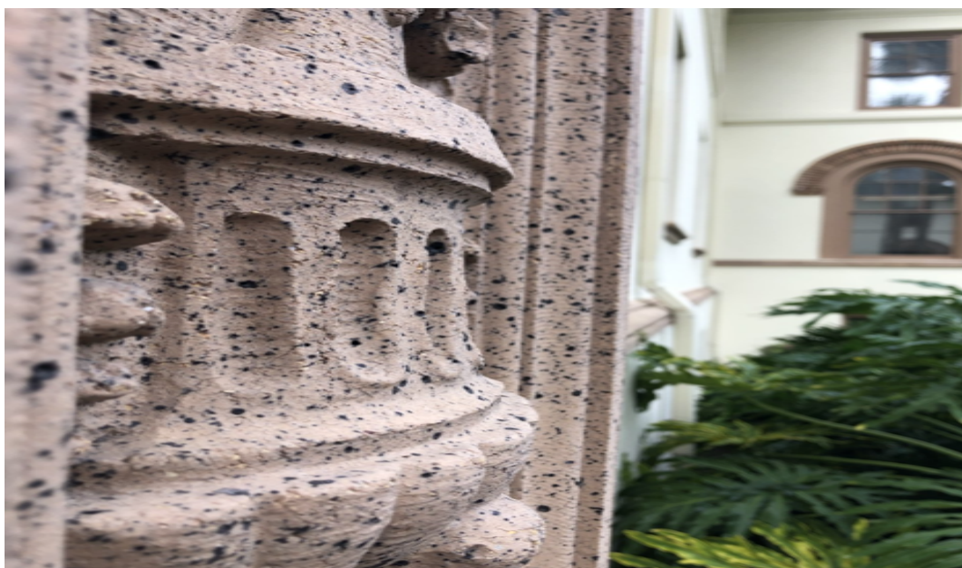
Flagler Hall Architectural Detail
