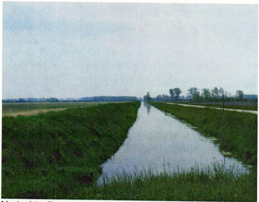
Much of the Township is well suited for farming, but requires extensive drainage, like this channel drain shown above.
