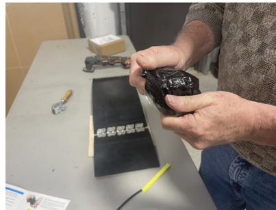
Mix by kneading and squashing the resin pack together until it starts to warm up (2-3 min).
