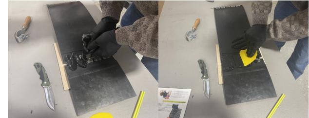
With clip joints, ensure that the FR1510 penetrates through all gaps between the pin and hinges. Use spatula or putty knife.
