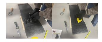
With clip joints, ensure that the FR1510 penetrates through all gaps between the pin and hinges. use spatula or putty knife.
