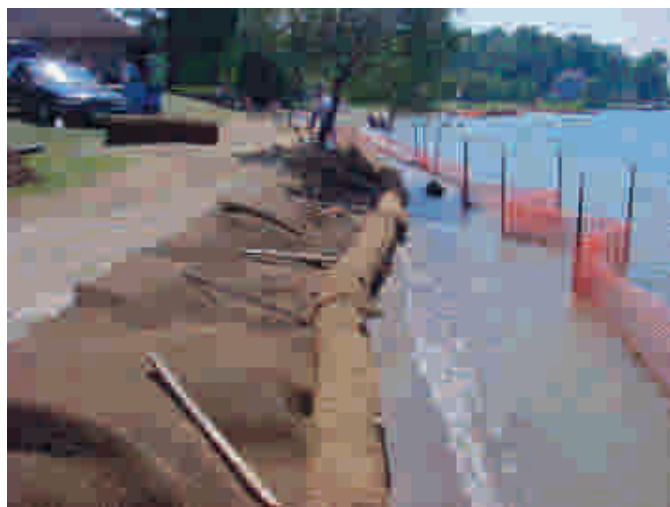
Installing coconut-fibre rolls
