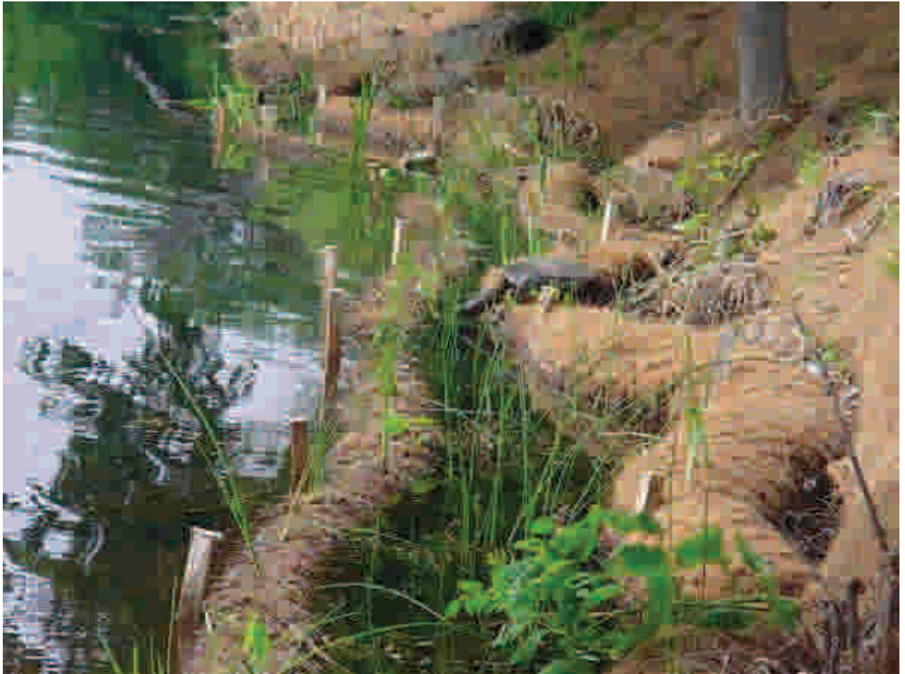
Coconut-fiber rolls installed
