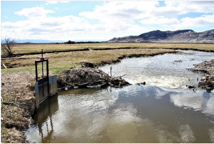
Headgate and diversion dam
