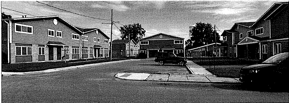
FIGURE 66: Existing Conditions of an Elkhart Housing Authority Parking Pod
