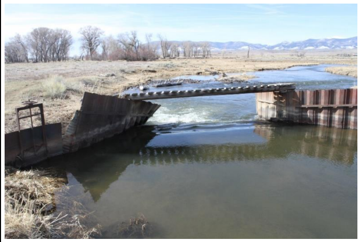
Headgate and diversion dam (on feeder ditch)
