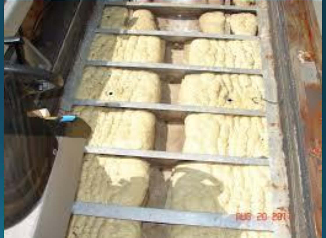
Adding floatation and structure between stringers
