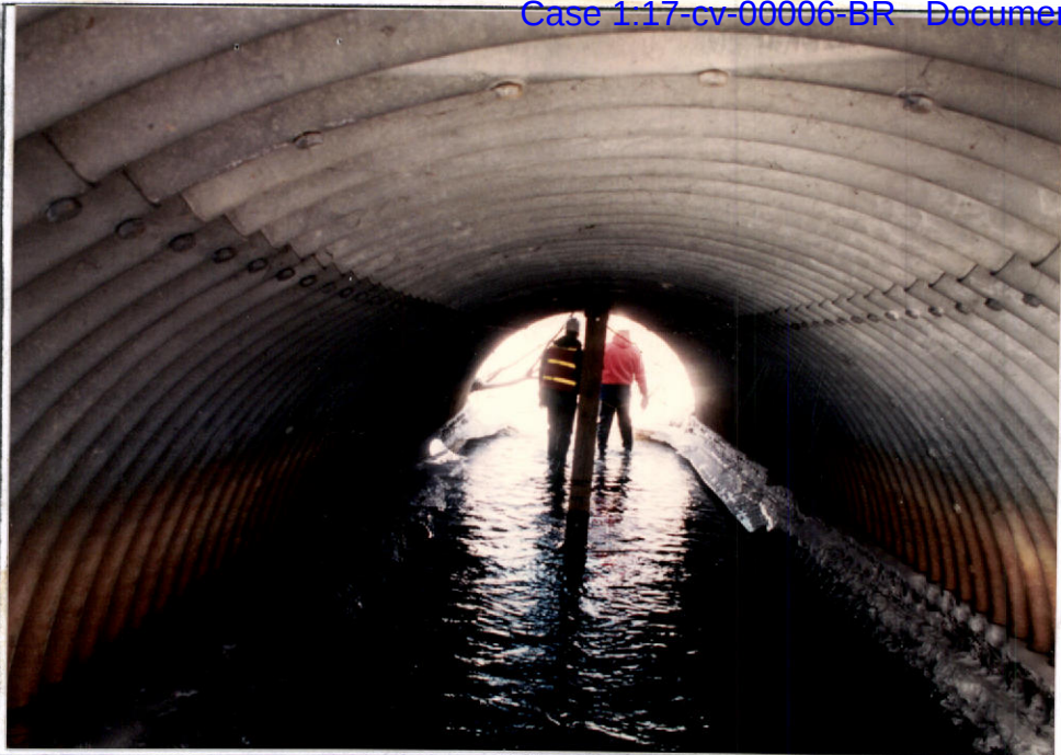
LOOKING DN. STREAM INTO STRUCTURE, CAMP PA
