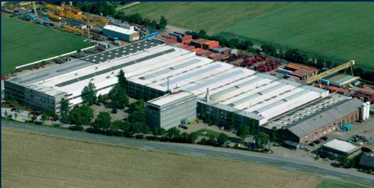
AUMUND headquarters in Rheinberg, Germany
