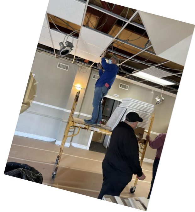
Sprucing up the Council
