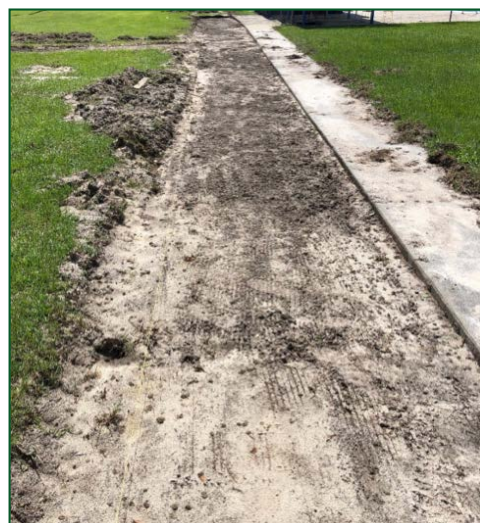
Forming of ADA Accessible Sidewalks
