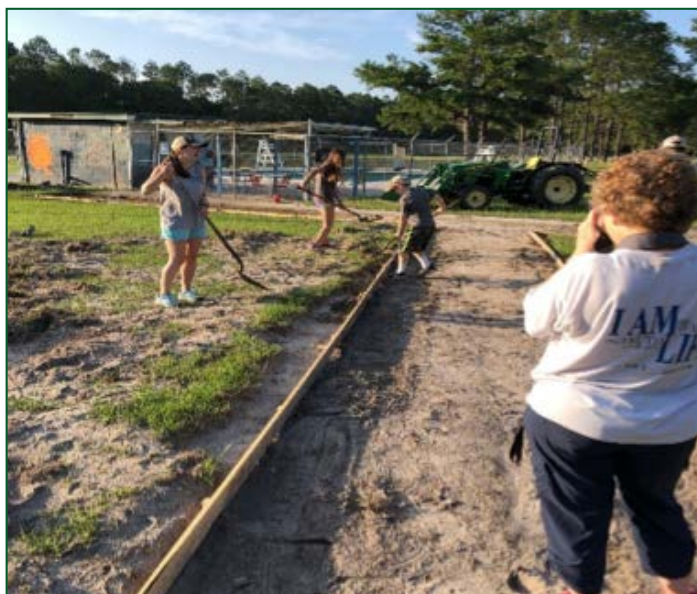
Lions and volunteers prepping sidewalk for concrete
