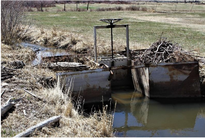
Headgate looking downstream
