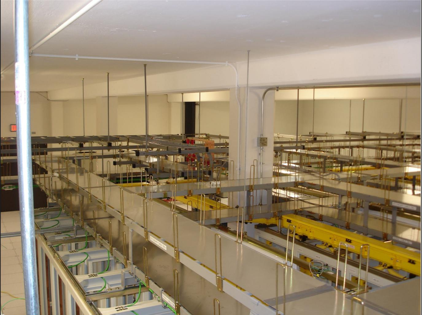
Showing build-out using 700 Series Frames, cable runway supports, cable rack and accessories as provided by Custom Cabinets & Racks
