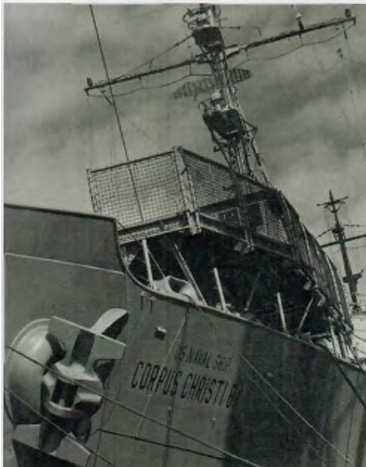
At its peak, the conversion of USS Albemarle , a World War II Navy sea-plane tender, to a helicopter repair depot renamed USNS Corpus Christi Bay involved 1,000 workers at the Charleston Naval Shipyard.
