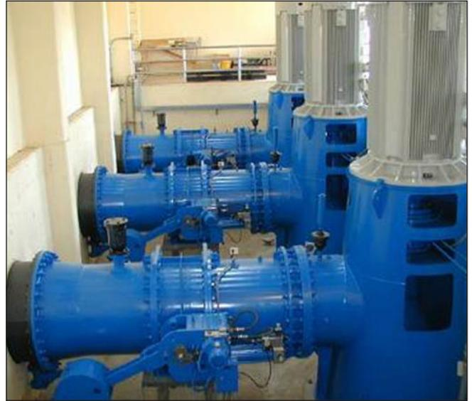
VAG EKN® 54" Butterfly Valve with HYsec for water supply at a plant in Poland.
