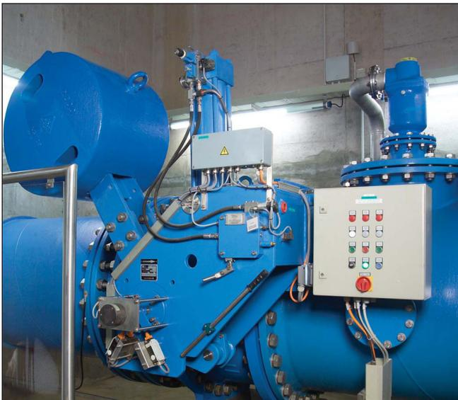
Vertical cylinder, anti clockwise closing
